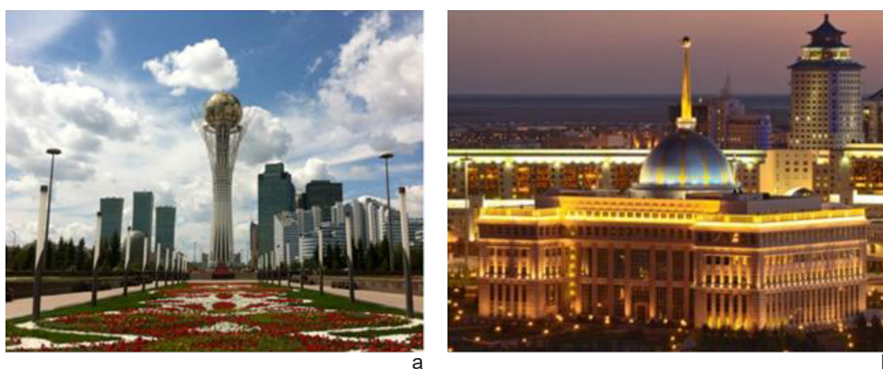
Fig. 3. Buildings of the new administrative center of Astana: a) “Astana-Baiterek” monument; b) Presidential Palace
