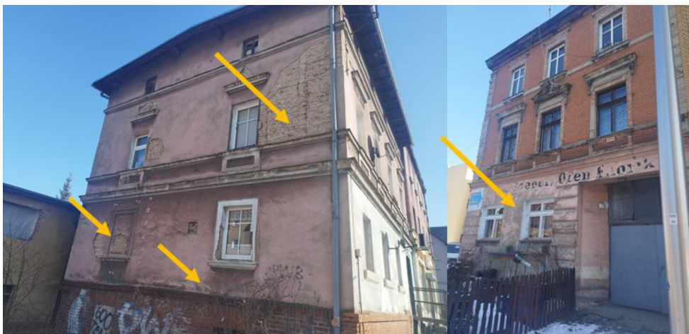
Fig. 5. Buildings requiring facade renovation, insulation, replacement of windows and doors, Jelenia Góra, Powstańców Wielkopolskich St. Source: own photography.
