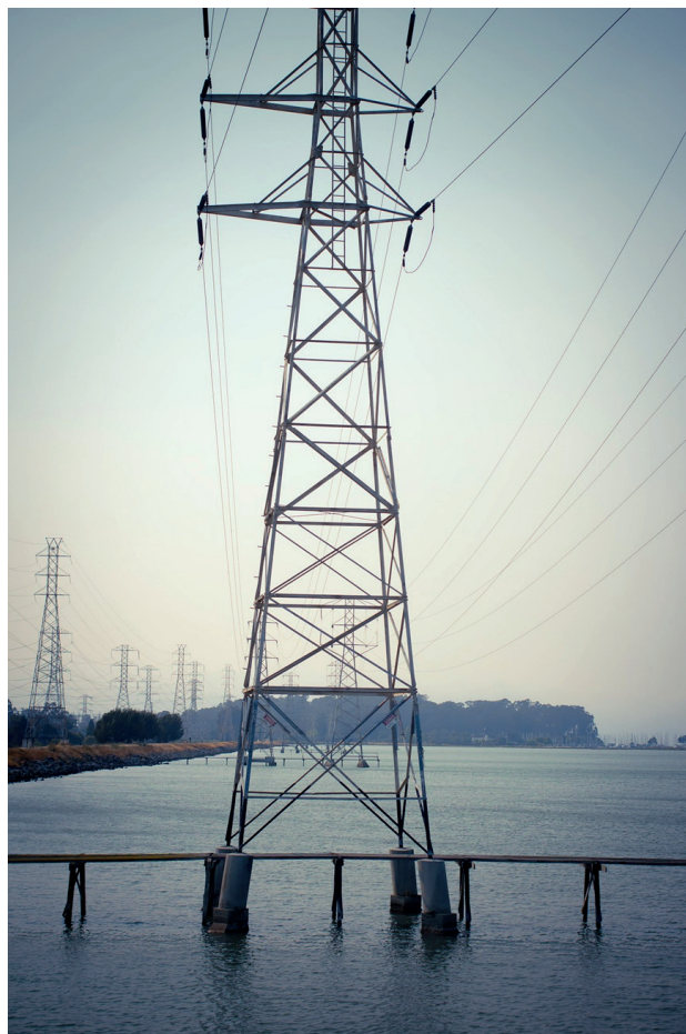
Fig. 2. Transmission towers on surface water supported on piled foundations
