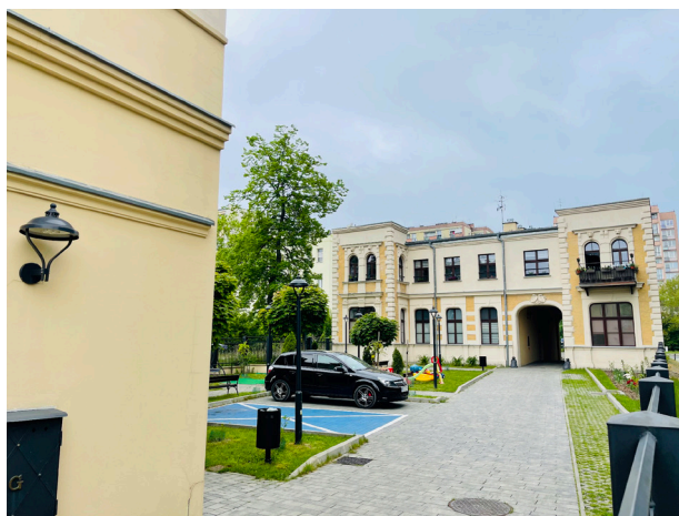
Fig. 3. Multigenerational house in Lodz from the side of the courtyard
